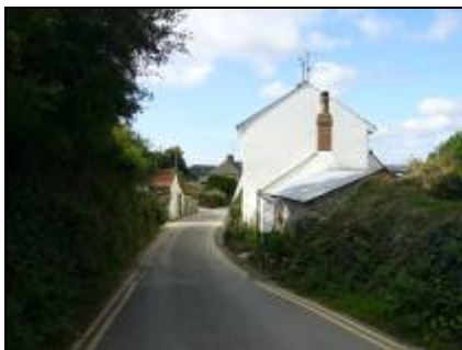
Strong arrival point to the settlement defined by the gable-end elevation of the Old Coastguard Cottages (6-9 Polkerris)
