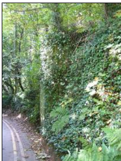
Remains of a footbridge crossing the approach road
