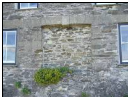
Common materials unify the built environment
