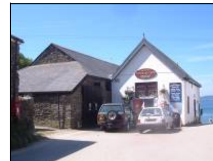
Fish cellar of 15 Polkerris, fronting onto The Square
