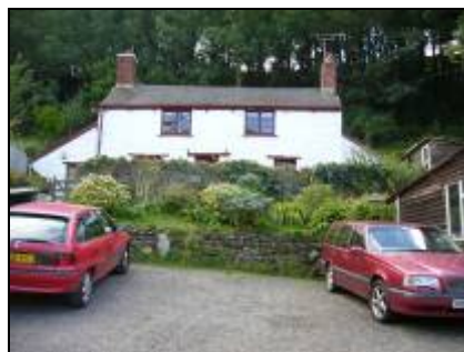
20 Polkerris, typical local detail with windows directly under eaves
