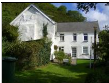
22-23 Polkerris, large gable-end stacks have been removed
