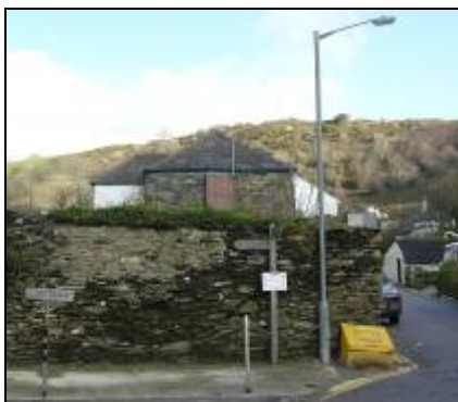
Parking control measures and the use of standard street furniture have a negative impact on the conservation area
