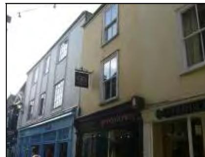
Flush windows are an indication of timber stud construction, Fore Street.
